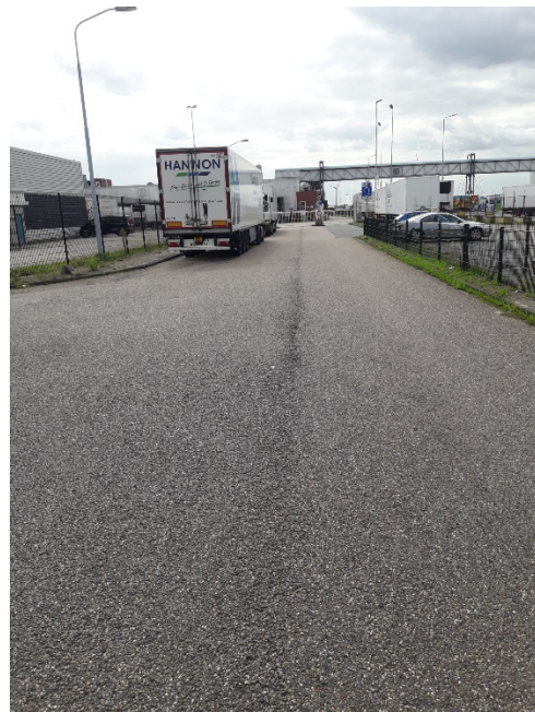
Foto 4, Scheurvorming en rafeling as
